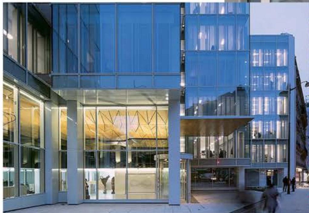
HQ "La Française", Boulevard Raspail, Paris Architect: Franklin Azzi, Paris – Photo: Luc Boegly, Paris Product: TOPPERFO Micro 2/2/0.5, Oak veneered
