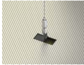
Solo Steel installation
